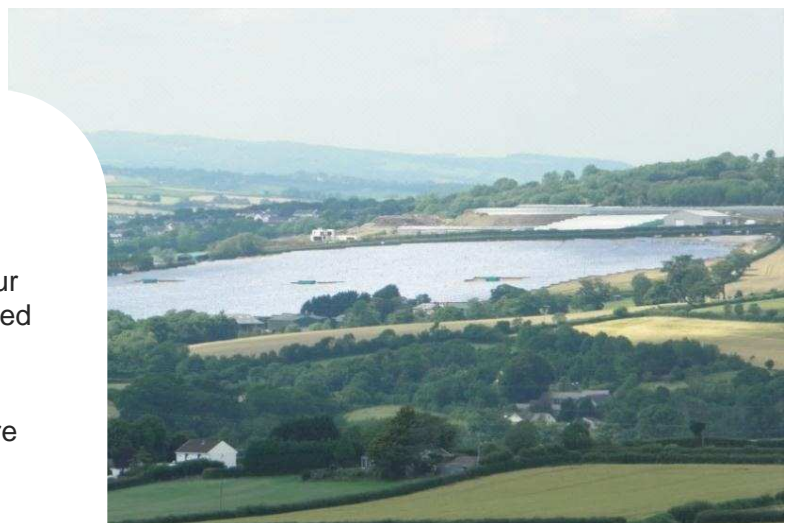
5 MWp group mounted PV in Cornwall, United Kingdom.
