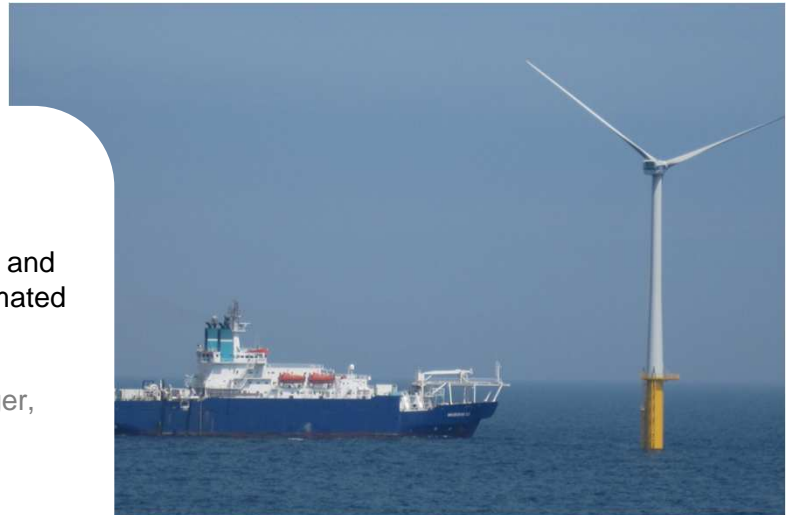
165 MW Offshore Wind Farm off the Coast of Belgium.
