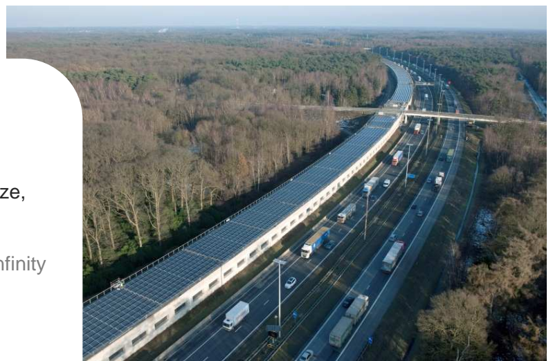
4MWp solar high speed train tunnel between Antwerp and Rotterdam.
